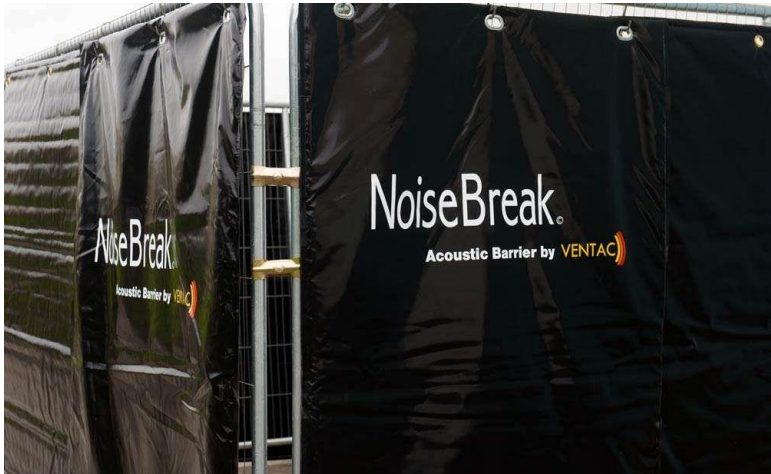
Figure 13.(a): Temporary construction noise barrier © Ventac
