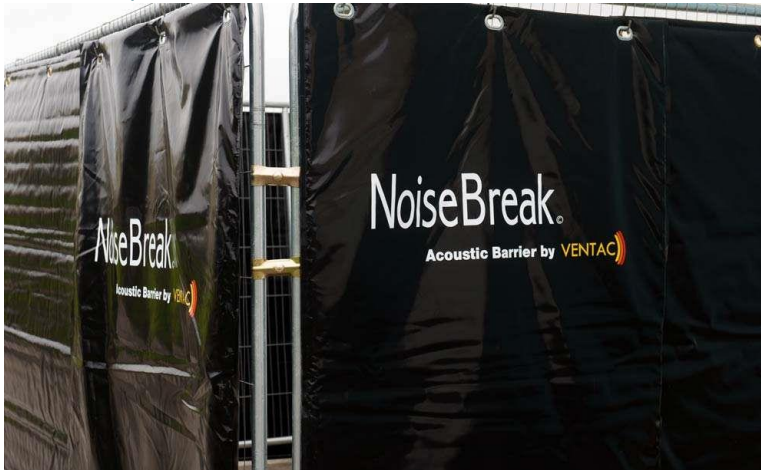
Figure 13.(a): Temporary construction noise barrier © Ventac
